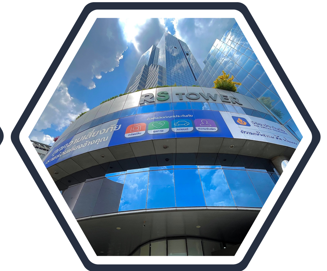
RS Tower, Rama 9 27th Floor
