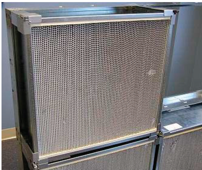
Figure 41: Properly Installed Filter Inside of the Frame
