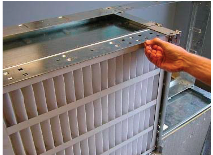
Figure 47: Installation of Prefilter into Frame
