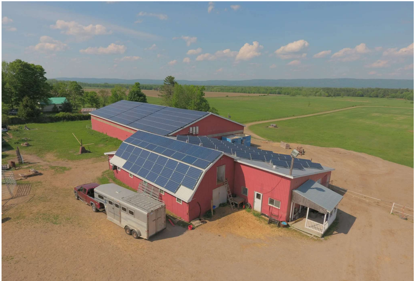
A solar project at Smith Farm in Dunrobin, Ont., near Ottawa, in 2016. Oil and gas companies are not spending profits to reduce emissions or switching to clean energy like solar. They should. Photo by iSolara
