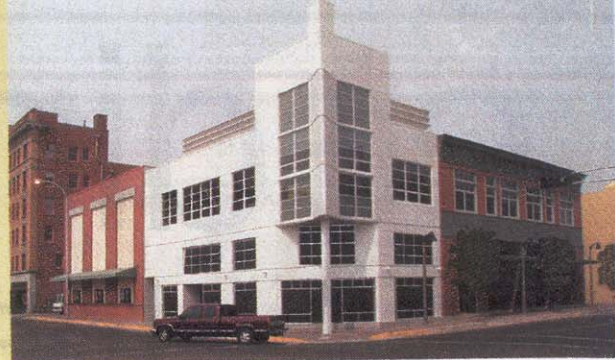
This retail and office building, by Moule & Polyzoides, gives prominence to an important corner and wraps a cinema's blank walls.
