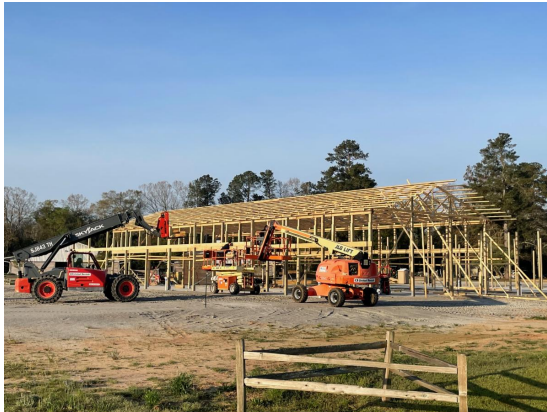
July 2022 Barn 17 Under Construction
