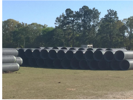
April 2015 Staging for Initial Construction
