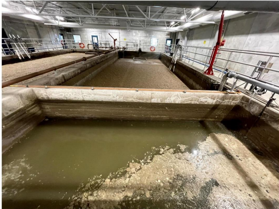
Figure 3: The same pre-react zone as Figure 2 but after a couple days of the Titus Twister running. Notice minimal amount of FOG.
