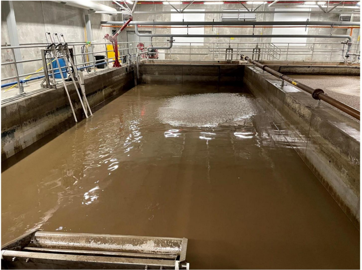
Figure 4: One of the basins after a month of the Titus Twister running. There is no foam on the surface showing just mixed liquor.
