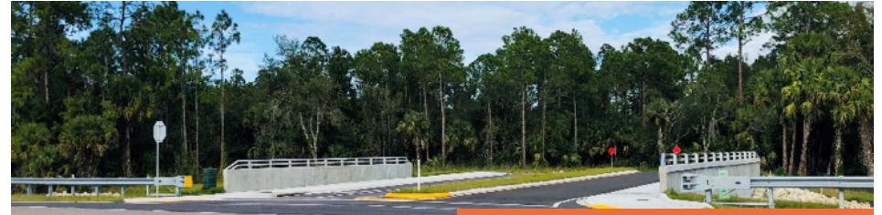
Kaicasa Bridge Entrance Complete
