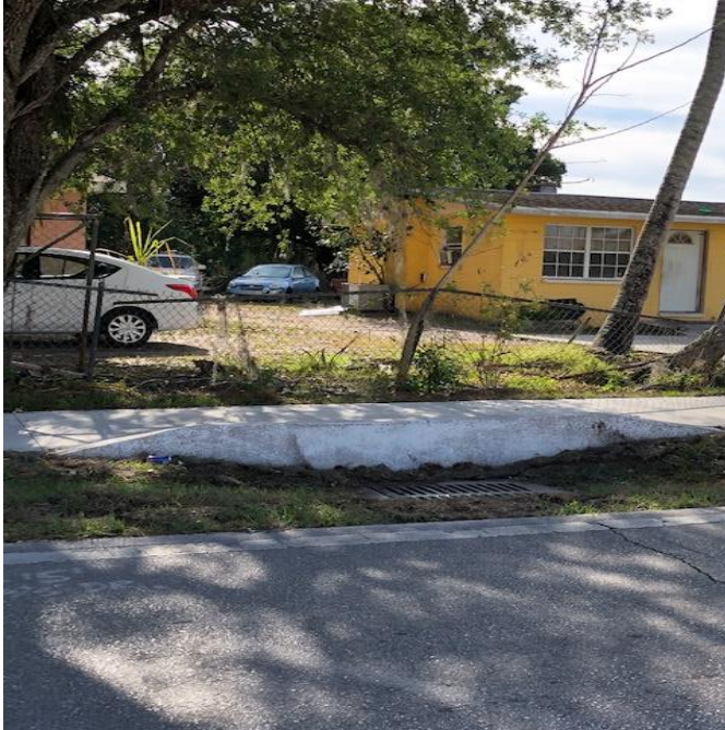
AFTER: Punch List completion of curbing with 3' transitions
