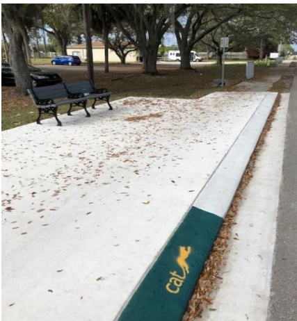
Roberts Senior Center Bus Station 2.19.21
