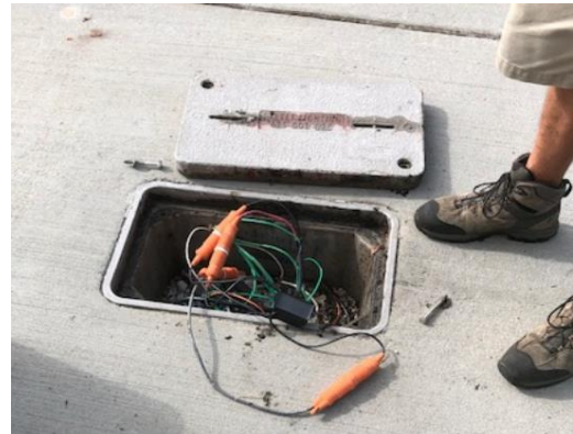
Inspection of the breakaway fuses and solid plugs. Standard detail plans show them in ground box– 4.12.21
