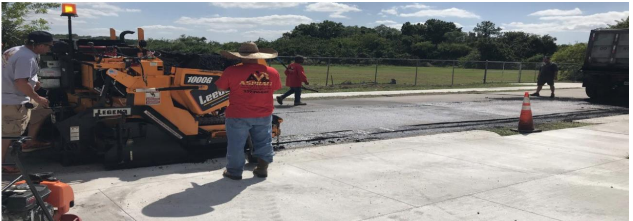
AFTER: Punch List completion of open cut on Carver
