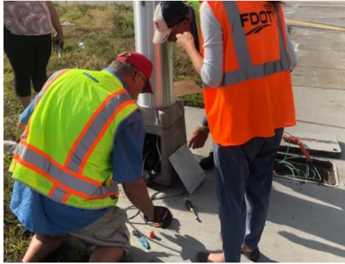
Inspection of the breakaway fuses and solid plugs. Standard detail plans show them in ground box– 4.12.21
