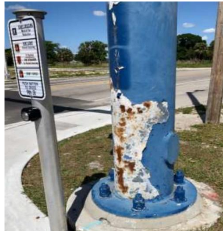
Signal Pole at Main St/9 th St 3.10.21
