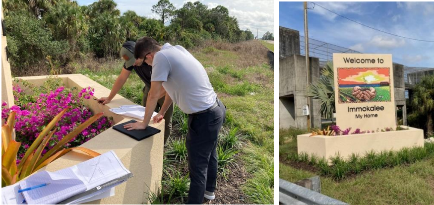
12.01.23 Walk-Through Inspection with Richard Chalupa, Q. Grandy Minor, and Jack Whittaker with Vctor Contracting
