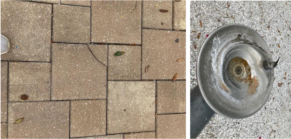
11.13.23 cracked paver and non-draining water fountain are being repaired
