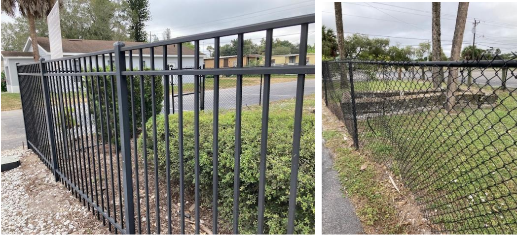
11.13.23 Historical Cemetery's fence maintenance and repairs
