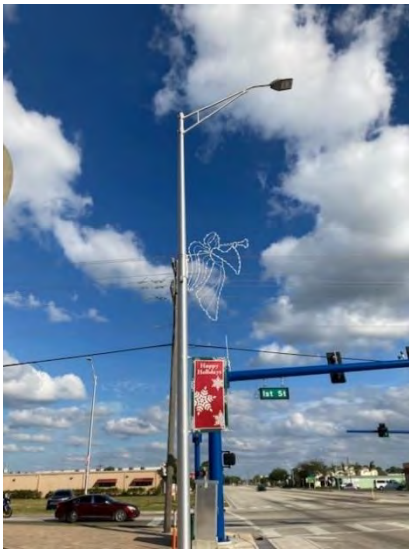
11.19.22 A&M installed the angels & banners
