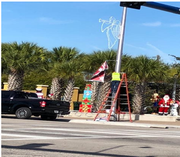
12.3.21 Installation of holiday banners by A&M
