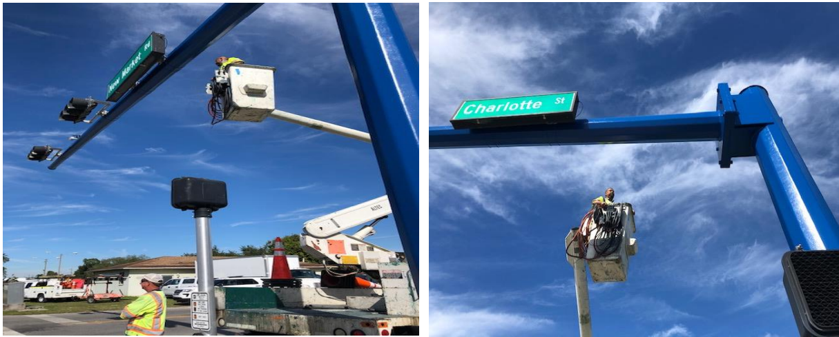
12.3.21 Inspection of painted poles at New Market/Charlotte
