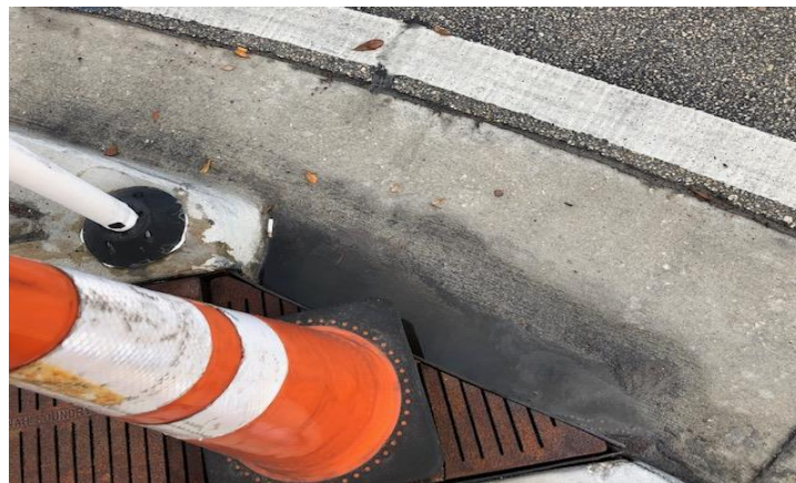
12.6.21 grate repaired at Main/S 4 th St
