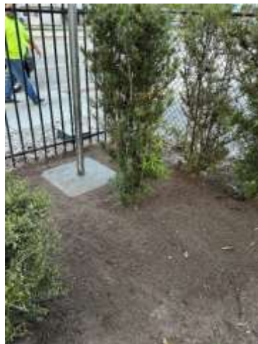
01.16.23 Signage repaired with concrete base
