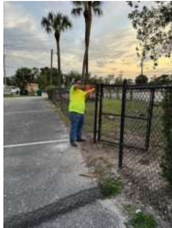
01.16.24 Gate repaired and gate now closes.
