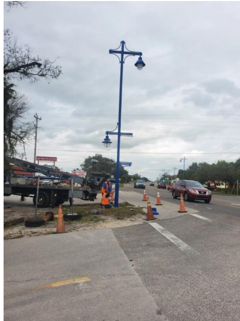
12.17.22 Installation of Pole #20
