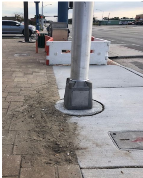
Zocalo new light pole and sidewalk 1.11.21
