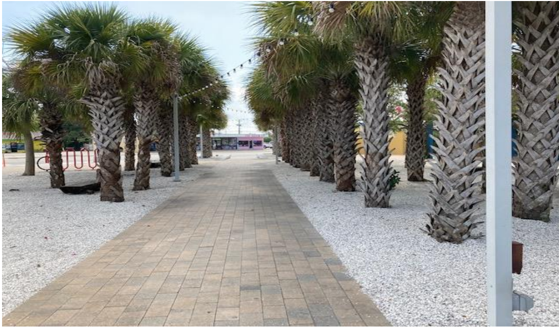
03.06.23 Overhead lights installation completed the Lighting Enhancement Project
