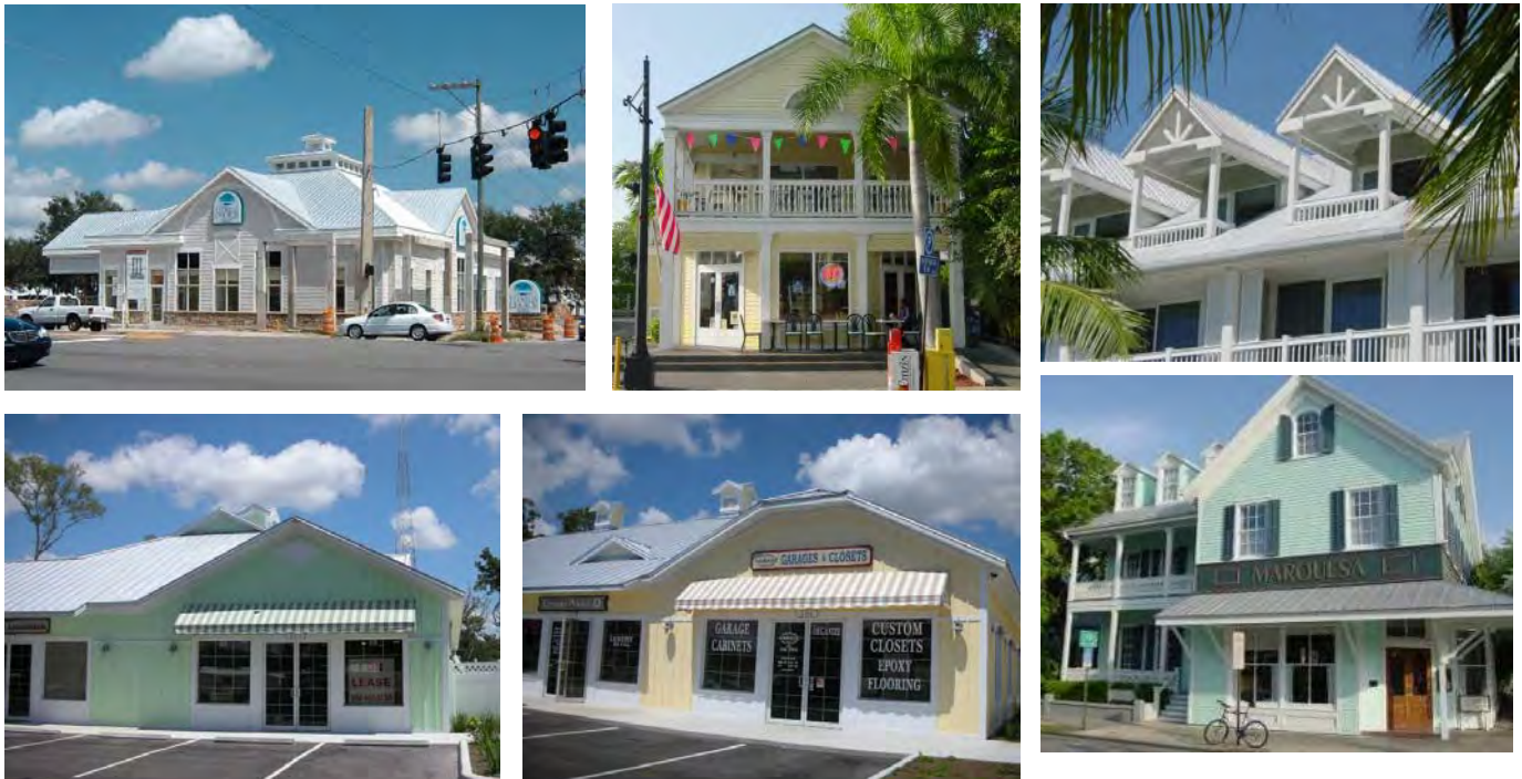
Examples of Frame Vernacular Buildings
