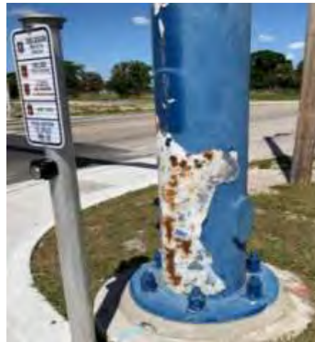
Signal Pole at Main St/9 th St 3.10.21
