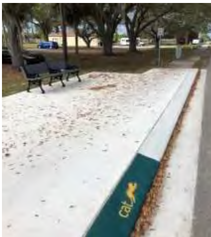
Roberts Senior Center Bus Station 2.19.21
