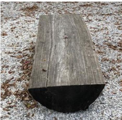
Current condition of wooden benches
