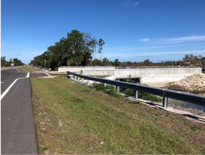
02.25.22 SR29 at entry bridge of Kaicasa project
