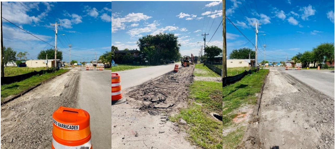
04.26.23 Area 1 - East Delaware Avenue Progress Photos
