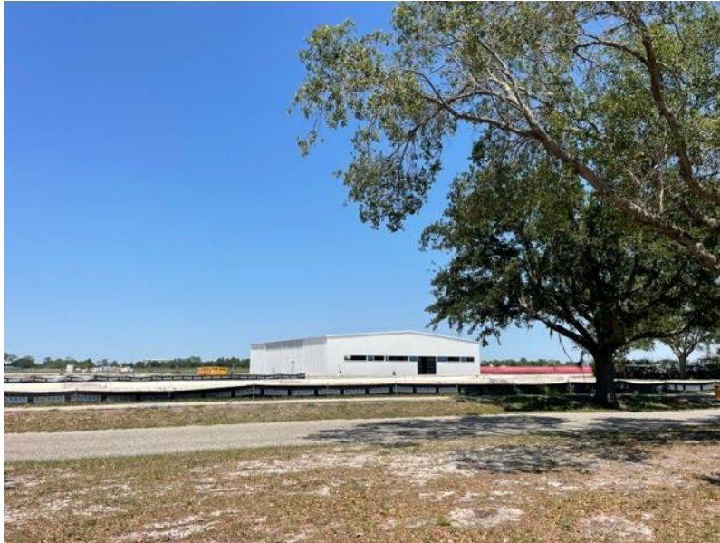
05.04.23 Construction of new Hanger
