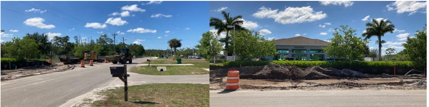
05.08.23 Area 1 - East Delaware Avenue Progress Photos
