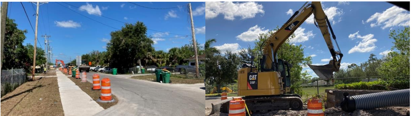
05.08.23 Area 1 - School Road Progress
