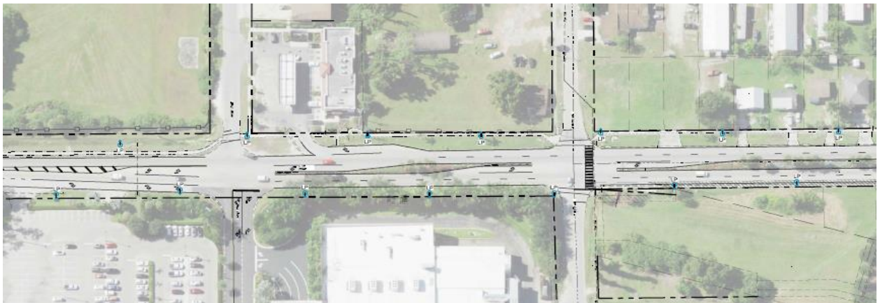
LCEC lights south of Casino on S 1 st St, DOT lights north of Casino on S 1 st S to Main St, and FDOT lights at the corner of Main St and S 1 st St
