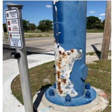
Signal Pole at Main St/9 th St 3.10.21
