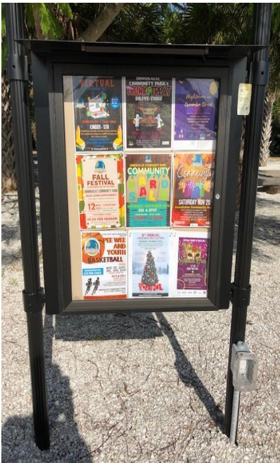
10.14.21 Kiosk awaiting lighting kit installation
