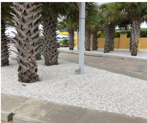
11.4.21 Zocalo Plaza new shell installation
