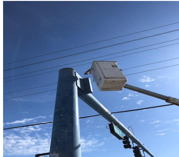
10.22.21 Main/1 st Pre-primer & paint inspection
