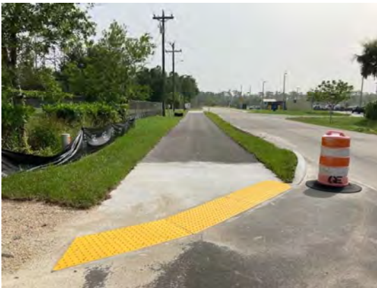
10.03.23 Improvements at Area 1 - South Park, School Dr
