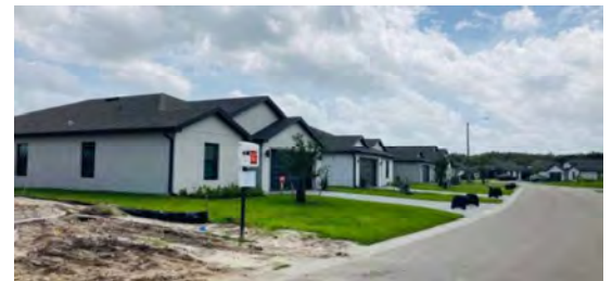
Construction on Arthur Street in Arrowhead Reserve Community.
