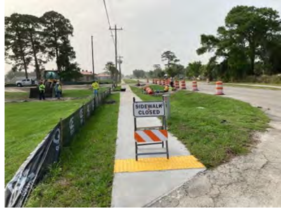
10.03.23 IWSD & QE Contractors working on Adams/Immokalee Dr
