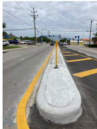
10.09.23 concrete/brick refilled medians.
