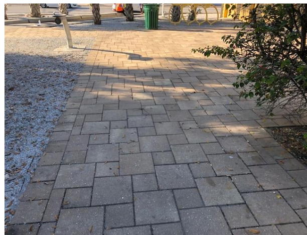
Repaired Pavers on 10.04.21
