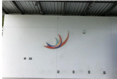
Bird of paradise installed 7.7.21.
