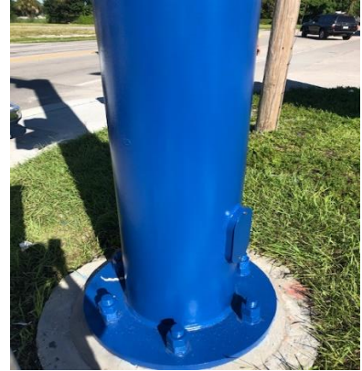
Blue primer applied to SE pole at 9 th St/Main 9.24.21 NE Signal Pole at Main St.9 th St N 10.13.21
