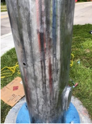
E Signal Pole 9.29.21
