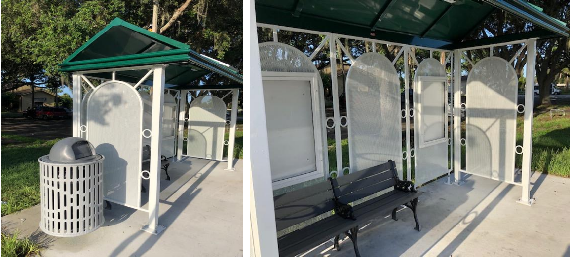
CAT Shelter Installed Robert's Senior Center 8.18.21
