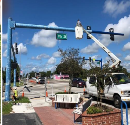
Blue primer applied to SE pole at 9 th St/Main 9.24.21 NE Signal Pole at Main St.9 th St N 10.13.21
