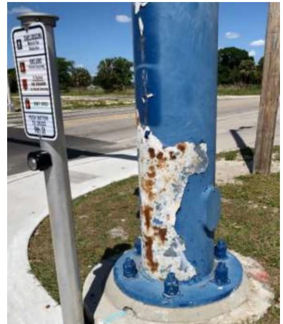
NE Signal Pole at Main St/9 th St N 3.10.21
