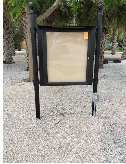
8.18.21 installed kiosk awaiting light kit
