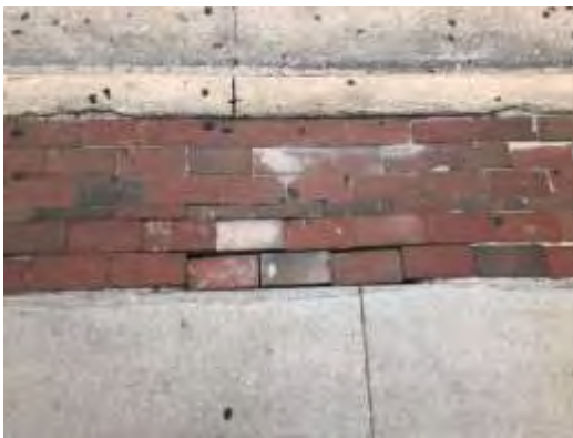
10.18.22 Azteca repaired & Handy/9 th St N also repaired
