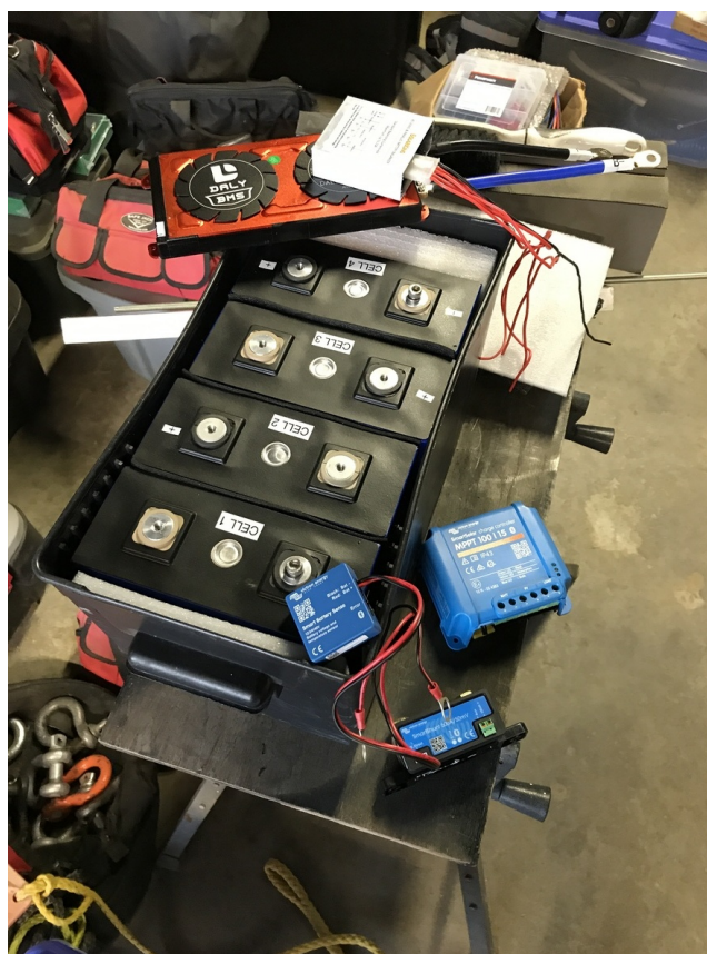
The beginnings of my battery box build.
