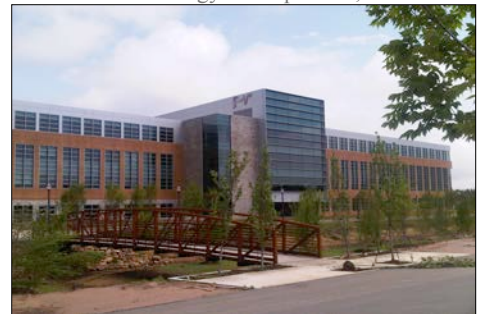
Southwestern Energy Headquarters, AR
