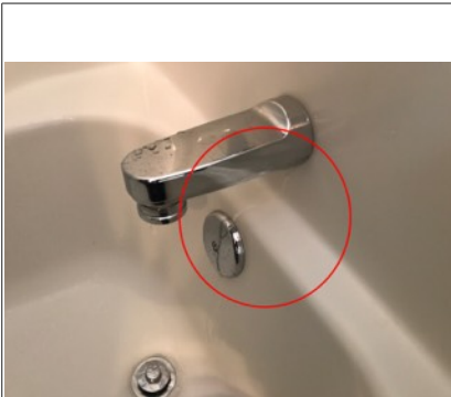
Tub spout leak.
