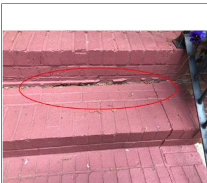
Spalling masonry.
