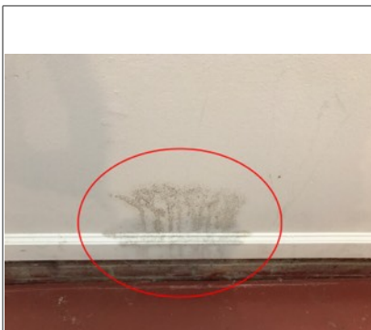
Surface mold staining on the front garage wall should ideally be cleaned.
