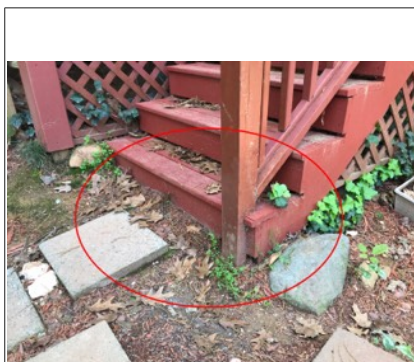
Wood to soil contact should be avoided on the rear deck steps.
