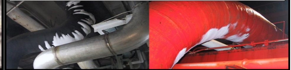
Crushed insulation material result in failure of Pipe support area Support Insulation areas are part of the pipes structural support. Ice Crushed insulation at those locations can cause very dangerous situations for pipe rupture caused by vibrations and friction to ships structure
