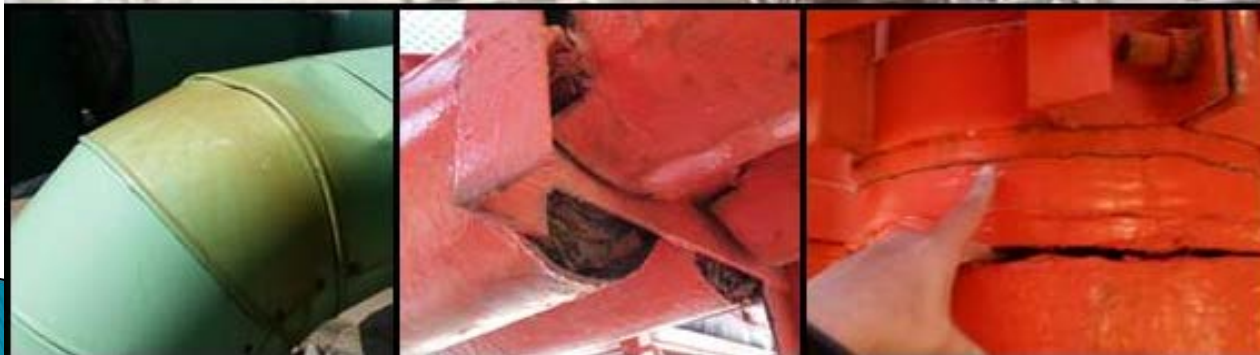
Crushed insulation material result in failure of Pipe support area Support Insulation areas are part of the pipes structural support. Ice Crushed insulation at those locations can cause very dangerous situations for pipe rupture caused by vibrations and friction to ships structure
