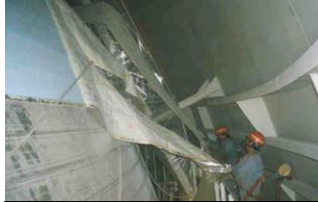
Peel off old outer barrier
