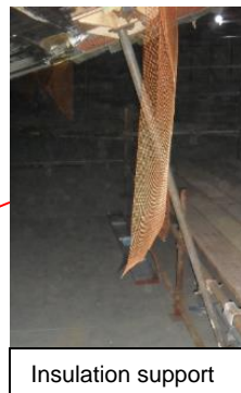
Strap Band to be released and insulation to be supported
