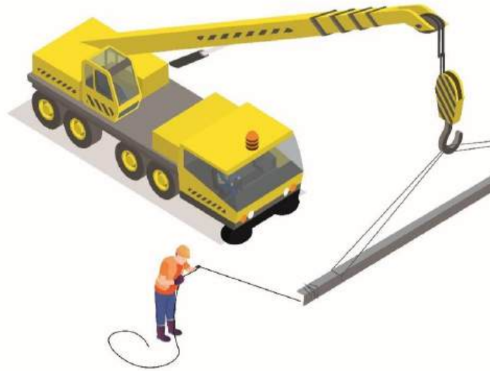
Fix tag lines to the end of the load before lifting
