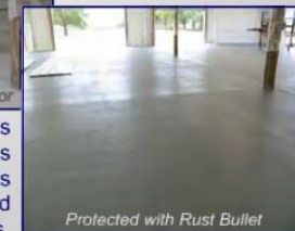
Protected with Rust Bullet
