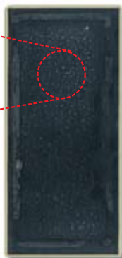
Tar Epoxy Resin Coating
