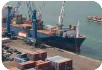
Slab port & runway
