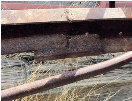
Welded frame extension
