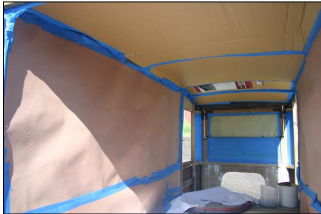
The interior cab area from rear of the driver entry door forward including the firewall will be spray painted black, so Tom has masked off the beautiful finished stained wood interior, the windshield and front corner glass from any overspray.
