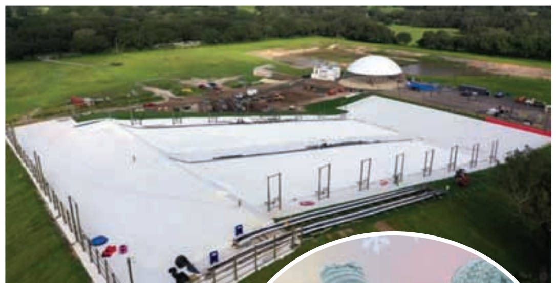
Above: Early-phase construction of the new snow park in Dade City.
