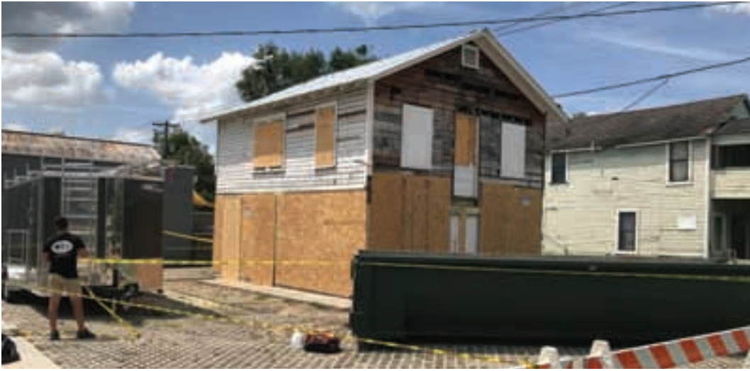
Kerns Family Construction is already on the job, just weeks after the proposal was approved by the Zephyrhills City Council. ANDY WARRENER
