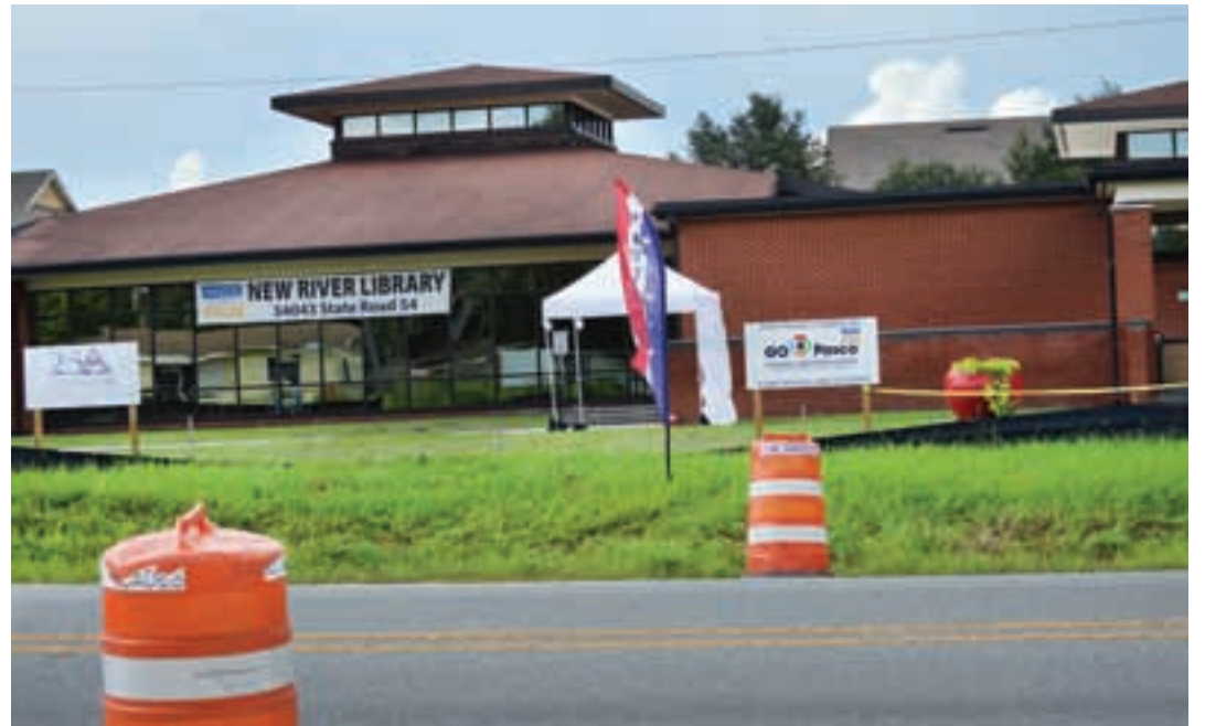
Renovations are under way at the New River Branch Library, which also served as a voting place during the recent elections. STEVE LEE
