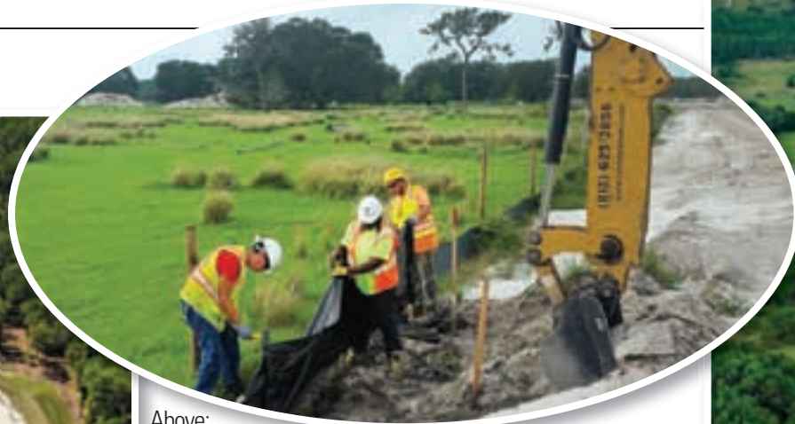
Above: Workers install a silt fence during construction of the SR 56 extension.
