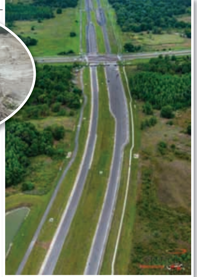
Above: A west-facing aerial shot of the SR 56 extension at the Meadow Pointe intersection, during early construction.
