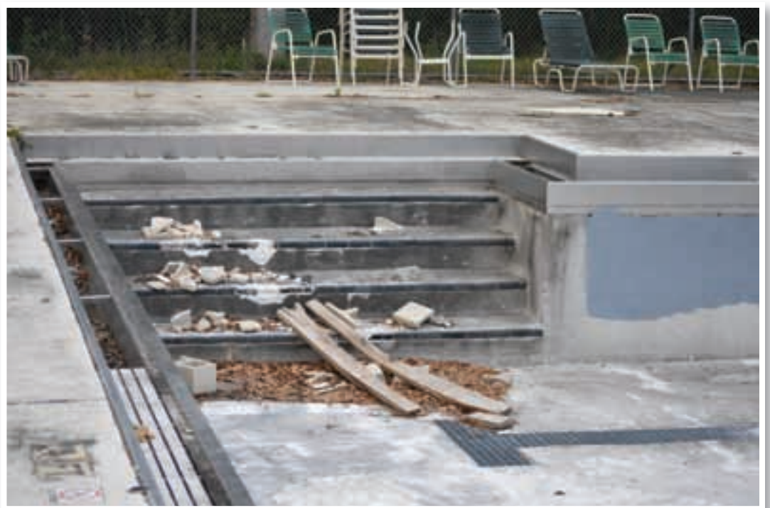
Above: What once was a nice pool and deck area is now in a state of disrepair. The entire facility will be demolished, although it has yet to be determined what will become of the Hercules property.
