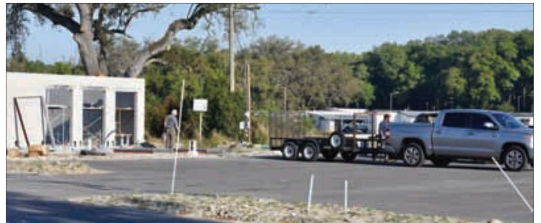
Workers showed up early one morning this week to continue building the structure of the new Veterans Affairs Clinic off Eiland Boulevard, just east of Fort King Road.
