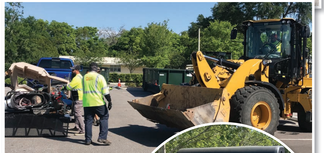
Above: A front end loader takes the dropped off items and deposits them in one of the 30-yard roll off dumpsters.
