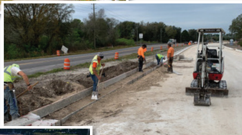
Below: Workers lay concrete curbing along the State Road 54 widening project.
