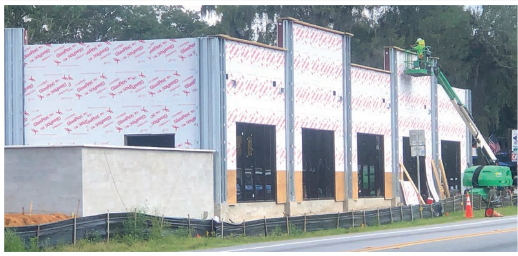
Left: The new Dollar Tree located on Gall Boulevard just up from another store of its kind.
