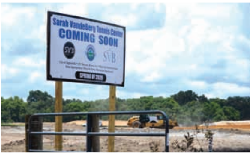
Left: Work has already begun as bulldozers clear land for the new Sarah Vandenberg Tennis Center.
