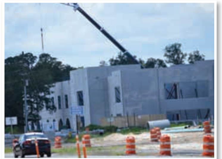
Above: Pinecrest Academy Wesley Chapel is being built along the State Road 54 corridor.
