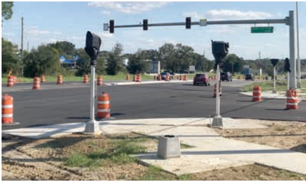
Above: The new mast arm signal and corresponding crosswalk signals at U.S. 301 and Medical Arts Court.
