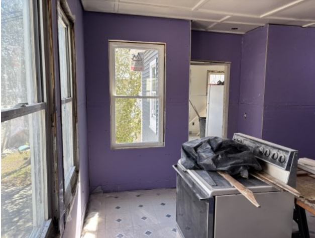
Unit 2's kitchen (second floor) with moisture resistant drywall on the walls. Plenty of sunshine in this room!
