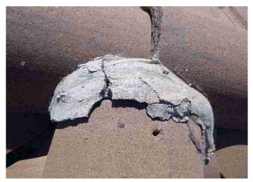
3.6 - Remove debris from roof surface. Debris on roof tiles can hold moisture longer and speed up deterioration of the roofing material. Also clean debris from roof wall transition flashing to prevent water from backing up under the roof tiles.
