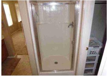
15.12 - The shower door seal is missing or damaged, and should be serviced. Monitor or repair as required.
