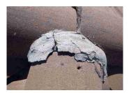
3.3 - Remove debris from roof surface. Debris on roof tiles can hold moisture longer and speed up deterioration of the roofing material. Also clean debris from roof wall transition flashing to prevent water from backing up under the roof tiles.
