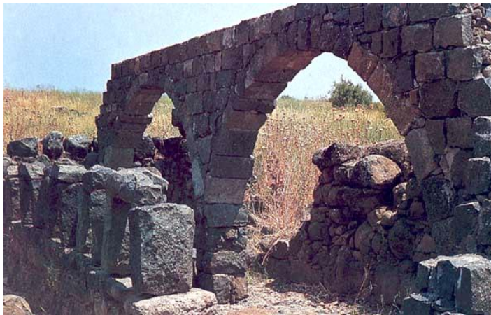
Arched walls in this domestic dwelling at Chorazin were typical of the area. The walls are constructed from basalt stone, a local volcanic rock that abounds in Galilee. Perhaps Joseph and Jesus did construction work with just such stones.
