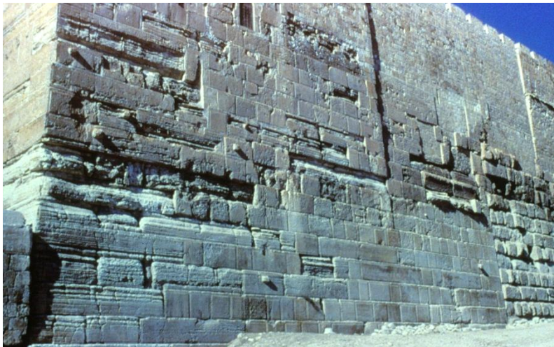
These ashlars, carefully shaped to fit snugly without a knife-blade space between, are the largest quarried stones in antiquity. The lower courses were laid by Herod, but the uppermost courses are post-Roman. To the right is a vertical straight joint, and scholars debate the age of the courses to the right of it, some suggesting a date as early as Solomon, others perhaps from Nehemiah's wall-building work (Ne. 6:15).
