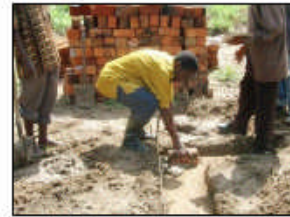
Laying the first foundation brick for the new Basoko church building
