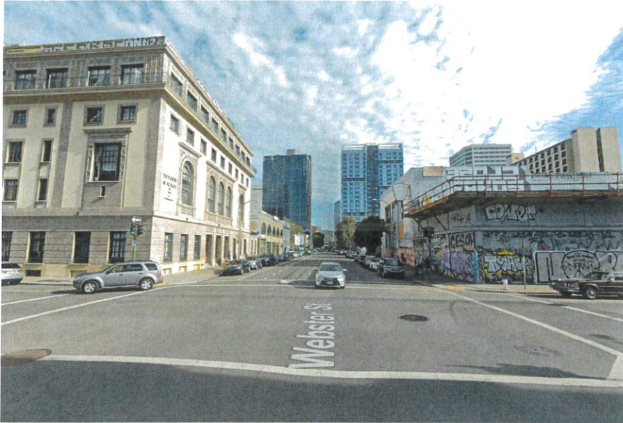
The YWCA on the left side with 1510 Webster Street on the right side of the image, courtesy Google Street View
