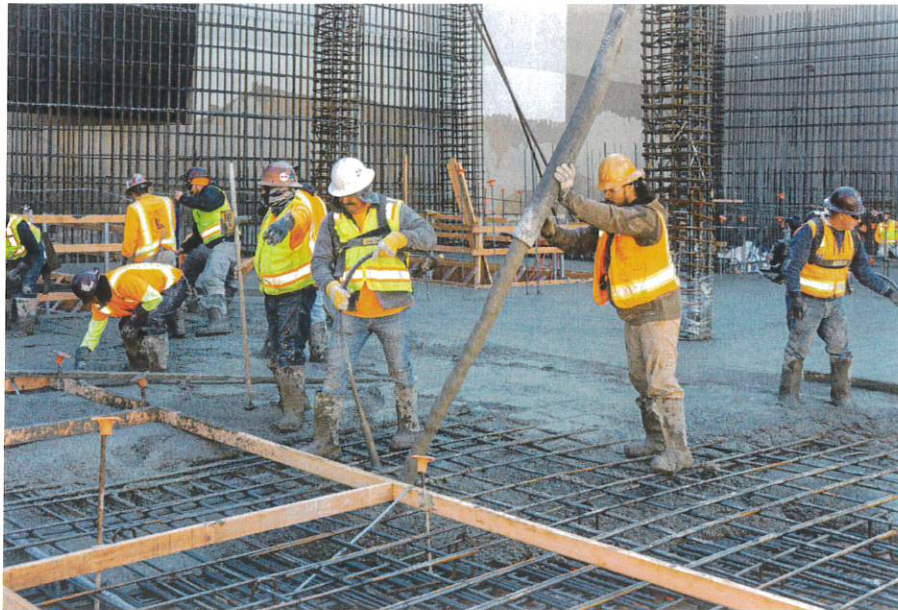
1900 Broadway concrete pour, image by author
